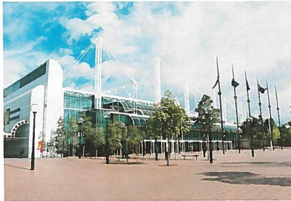
The impressive glass-fronted facade of Sydney Exhibition Centre.
